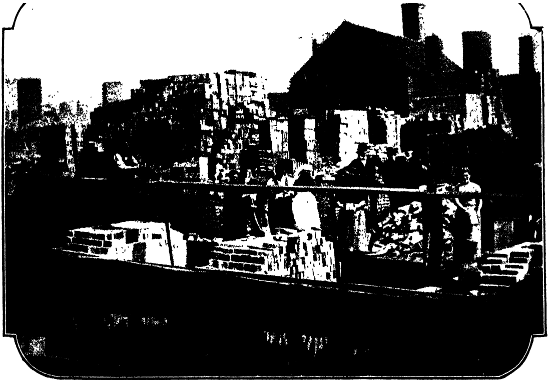
WOMEN BRICKMAKERS LOADING BARGES.
